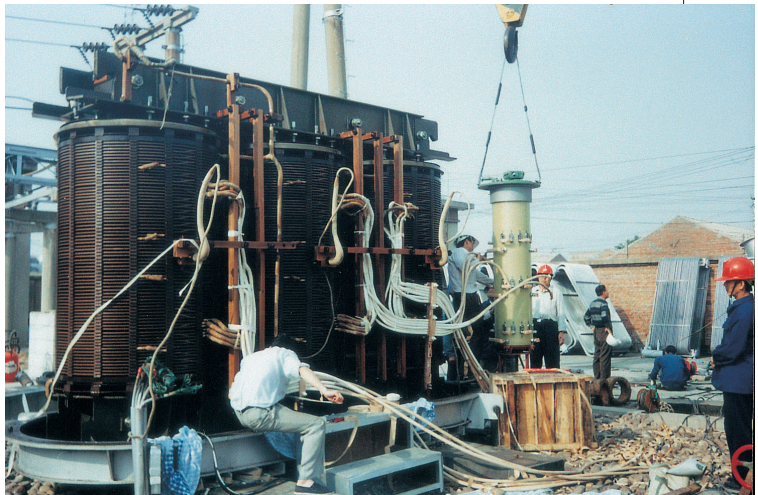
Leads connection during the retrofit of OCTC to OLTC
